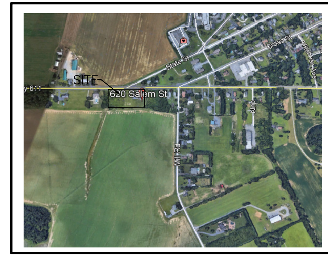
AERIAL PHOTOGRAPH N.T.S.
